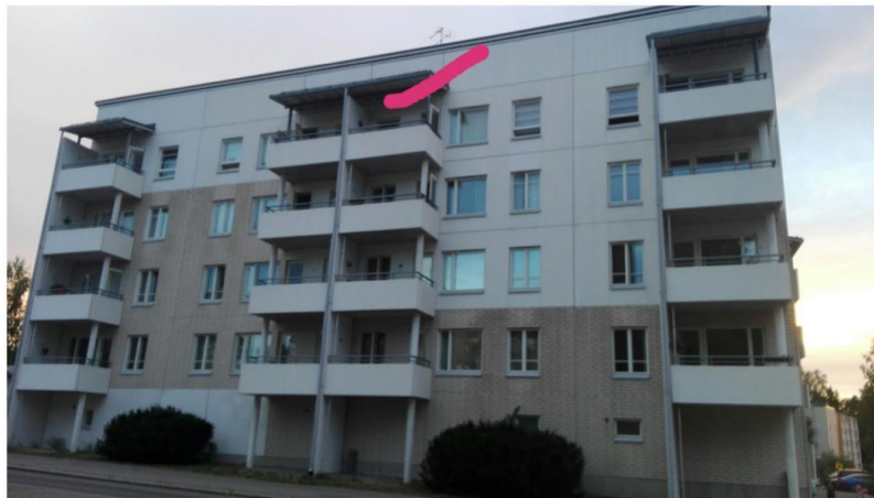
Figure 54. The balcony from which harmful items were thrown.
